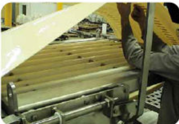
Belt repaired on site.
